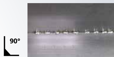
Corner spot welding thickness 0,6 mm
