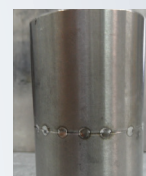
Pipe butt weld Ø 31.75 x 2 mm
